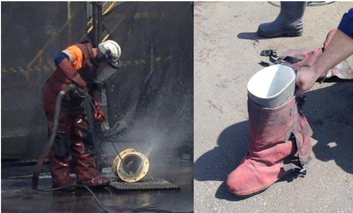
Personal protective equipment. Left: Worker using high-pressure water jetting equipment while wearing appropriate face shield, blast suit, protective gloves, and boots with covering foot shield. Right: Protective boot and covering foot shield.
