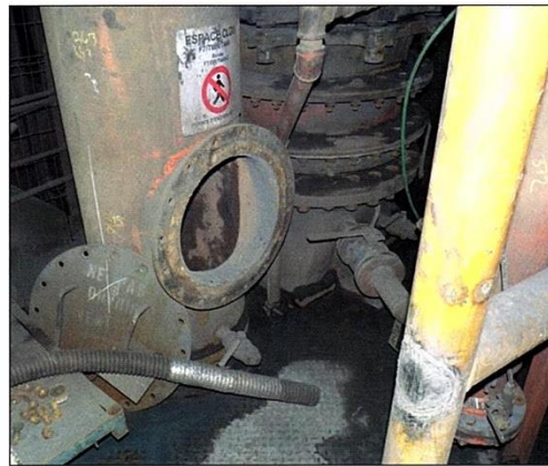
Figure 1. Access opening for cleaning
